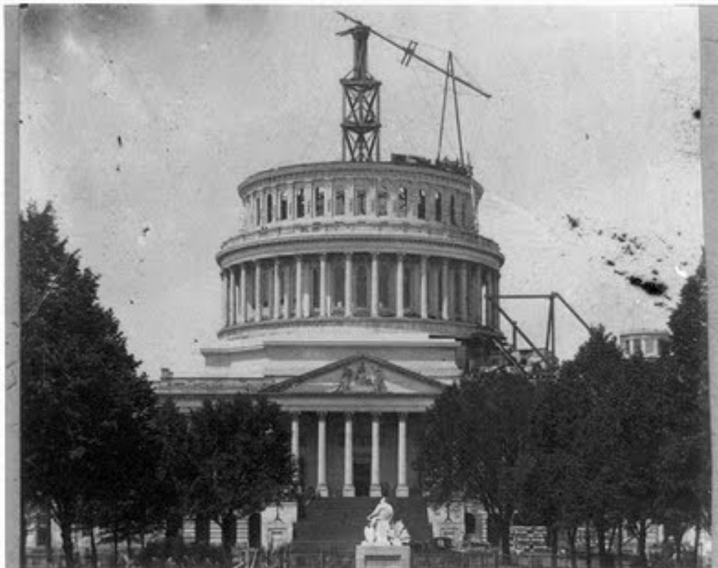
The U.S. Capitol under construction, May 1861 ( Library of Congress )
